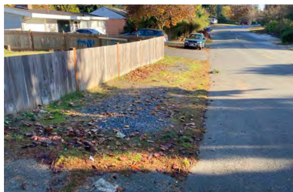
The neighborhood has many gravel ROW areas that could be retrofitted for infiltration.
