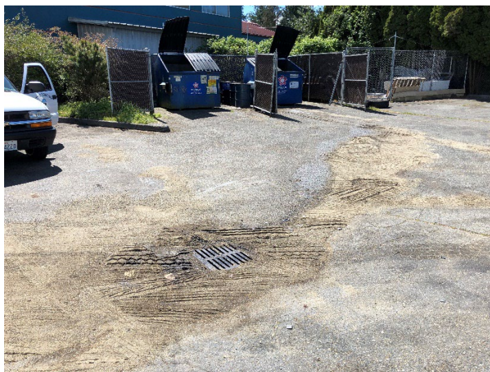
Illicit discharge next to commercial dumpster enclosure.
