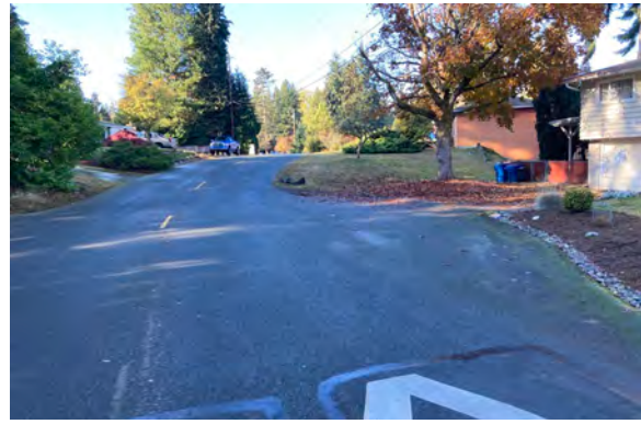
Section of 191st St SW with excess pavement that could be removed and retrofitted with bioretention.
